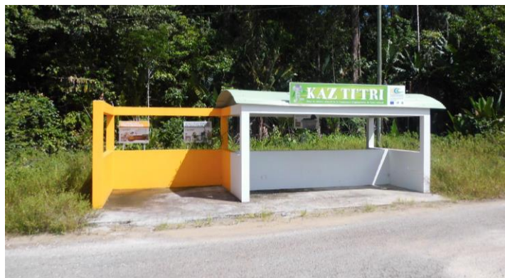
Photo 1 : Kaz Ti'Tri "MIMOSA" (zone ENC/DV + zone BACS)
